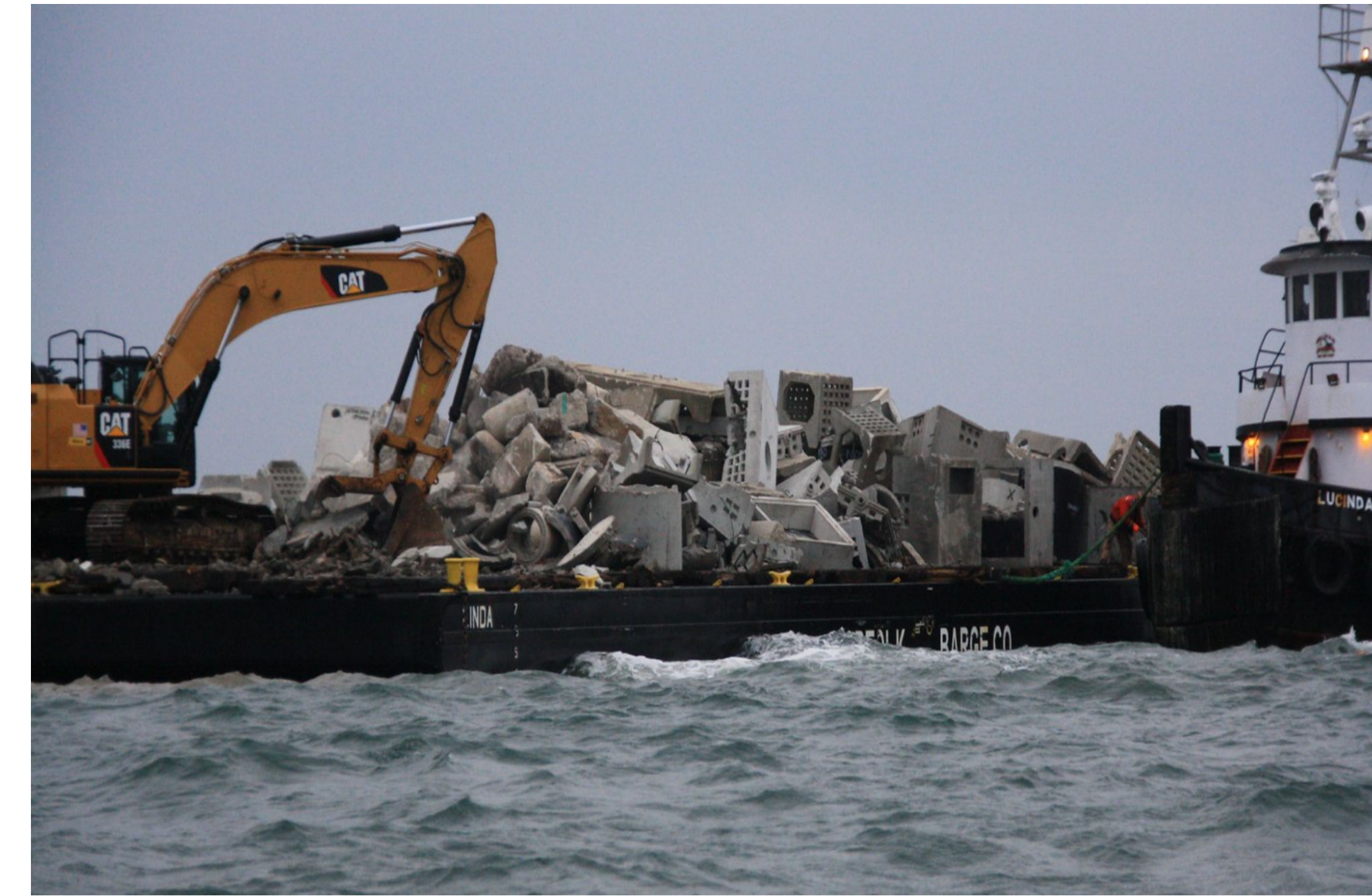
Construction materials used to make artificial reefs:
