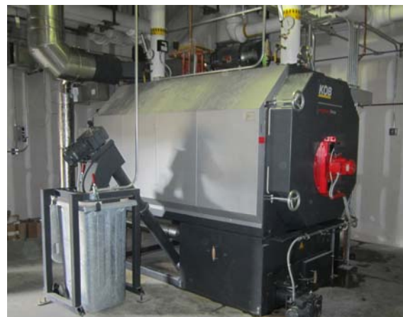
Wood pellet boiler
