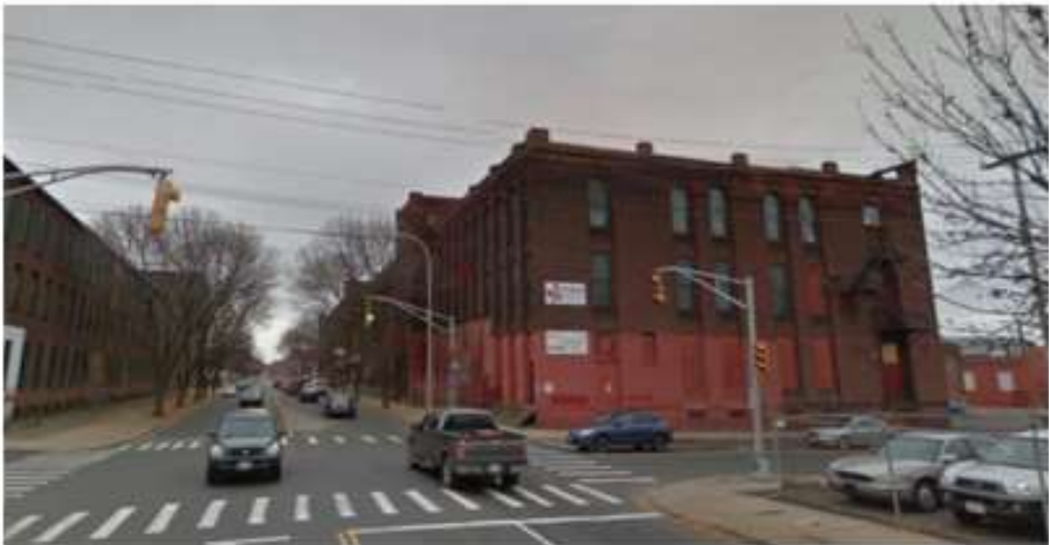
South west view
