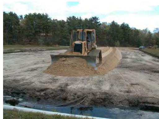
Fig. 1. (Top) Scraping and removing established vines. (Bottom) Applying a thick uniform layer of sand prior to planting. Photos courtesy H. Sandler.
