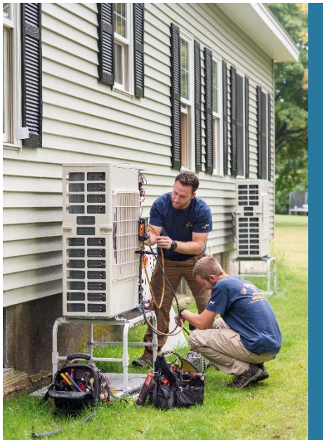
Picture 5. Two HVAC Technicians Installing a Heat Pump
