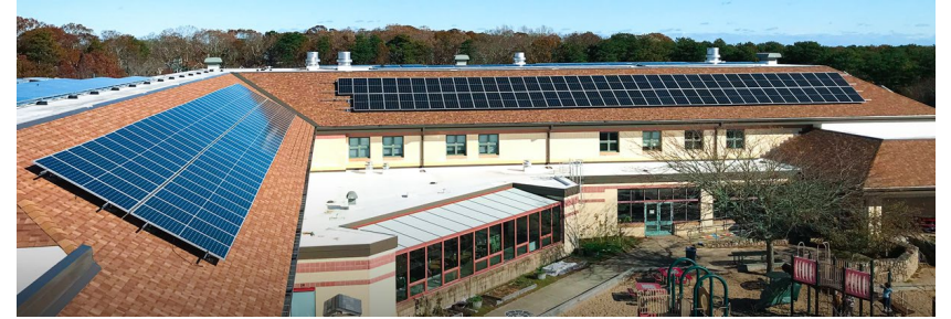
Oak Bluffs Elementary School Roof & BESS
