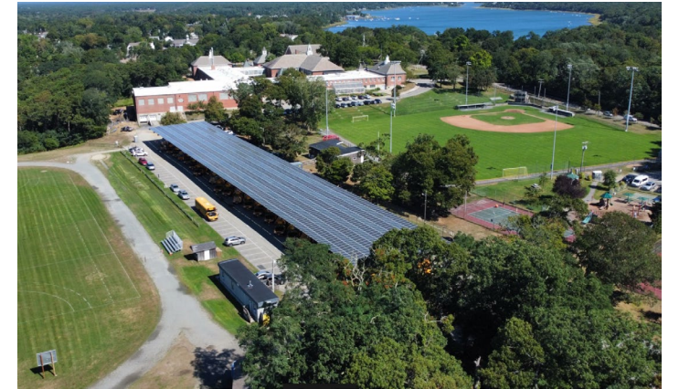
Nauset Regional Middle School Canopy & BESS
