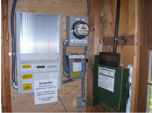
An inverter is needed to convert the DC power generated to AC power to feed the power grid or for collection operate equipment.
