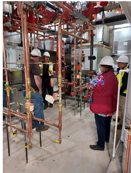
Inside the new mechanical room
