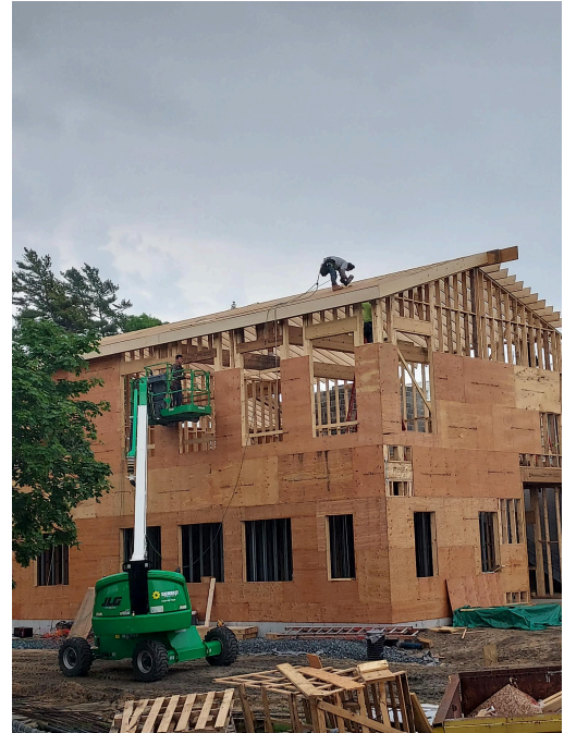
Framing the new building
