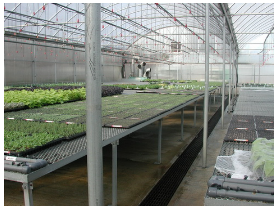
Heated Bench System for Propagation in Gutter-connected Greenhouse
