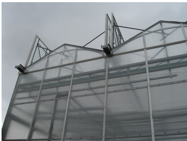
Rainwater Collection System
